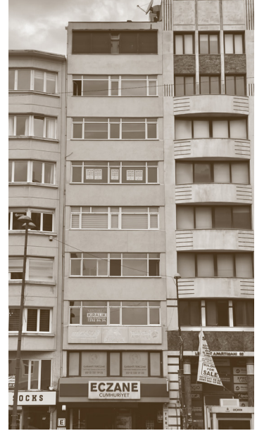
The building on Cumhuriyet Avenue, formerly No. 47, now No. 87. (Photo: Can Candan)
