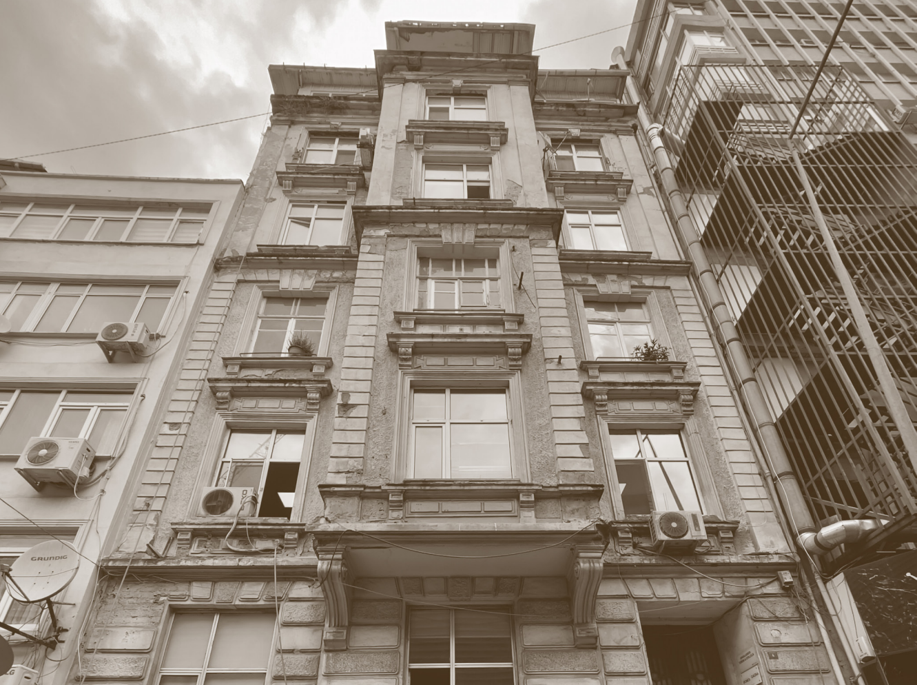
Elmadağ Avenue, former Nomiko Apartment. (Photo: Can Candan)
